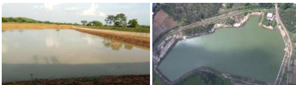
Figure 5: Reservoir construction under Jal Tirtha in West Bengal
